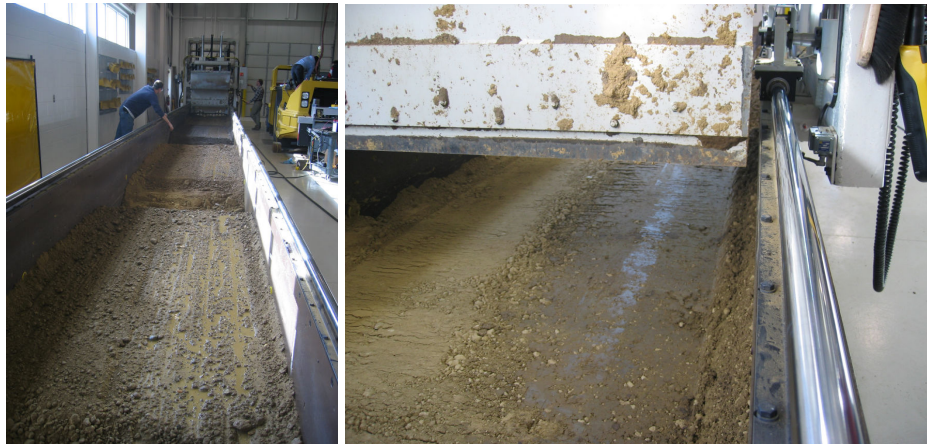
(26m, 26n) Preparation of wet and dry sides of the trench
