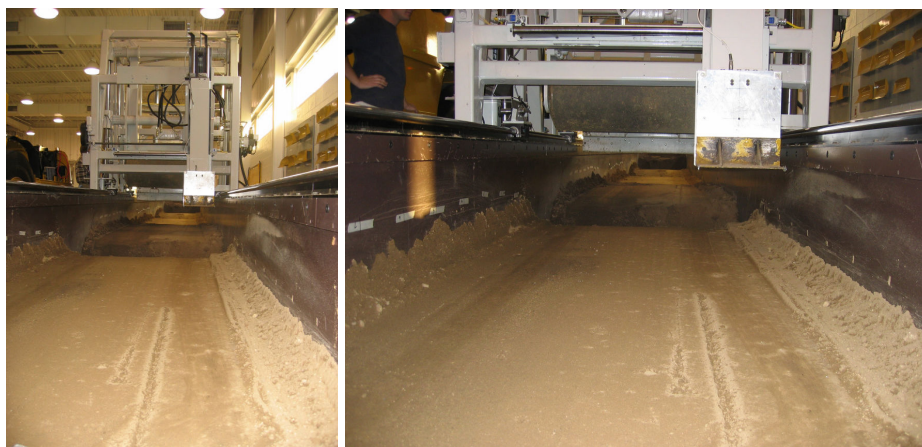
(26k,26 l) Wet and dry sides of the trench, being compacted thoroughly
